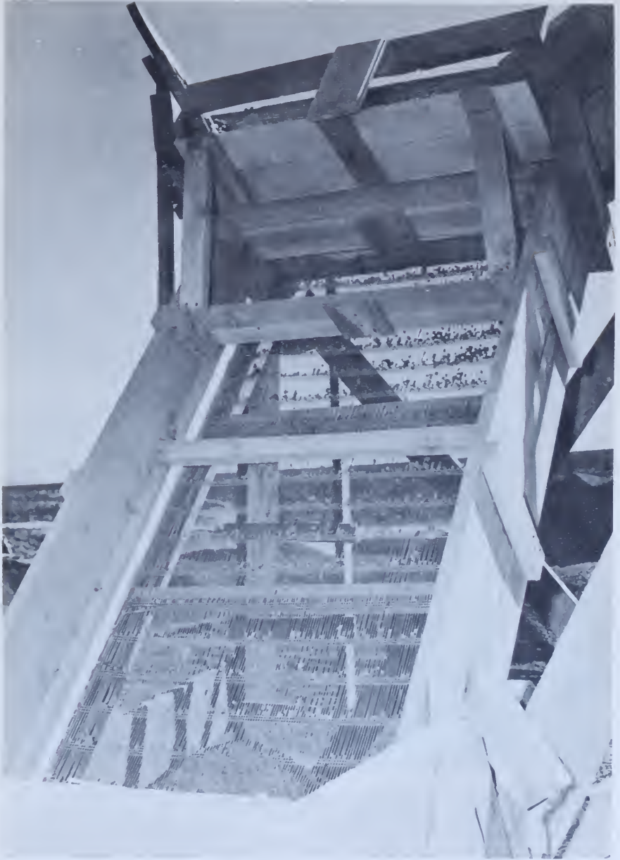
Figure 87.—Stationary screen with 3/16-inch by 4-inch slotted openings for finish screening coarse aggregate used on the Columbia Basin project, Washington. Note pile of undersize material visible through screen. CB-3702-4.
